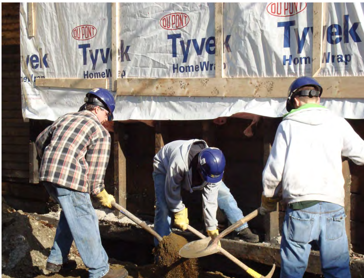
Pictured above are former Train for Trades participants digging at a worksite.
